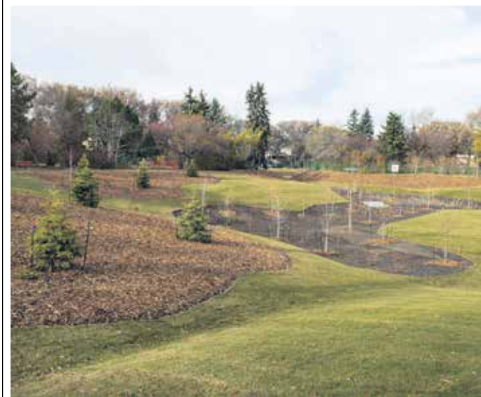
A recently completed dry pond in the neighbourhood of Parkallen in Edmonton is an example of the range of measures that can contribute to stormwater mitigation. SUPPLIED
